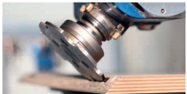
Cutting recesses for connecting fittings
