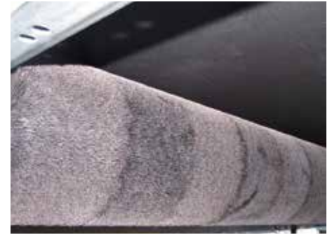
Belt cleaning equipment
